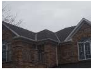
Pic. 2: Updated roof covering
