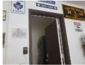
Pic. 7: No auto closer on garage entry door
