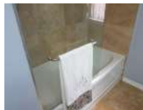
Pic. 19: 2 nd floor bath
