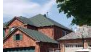
Pic. 3: Updated roof covering
