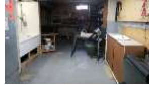
Pic. 39: Unfinished basement area
