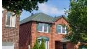
Pic. 2: Updated roof covering
