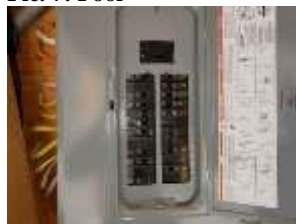
Pic. 11: 100 amp breaker panel
