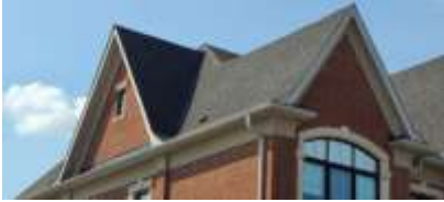
Pic. 4: Roof covering
