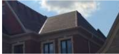
Pic. 2: Roof covering
