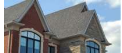
Pic. 3: Roof covering
