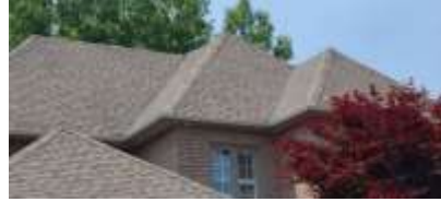
Pic. 2: U[dated roof covering
