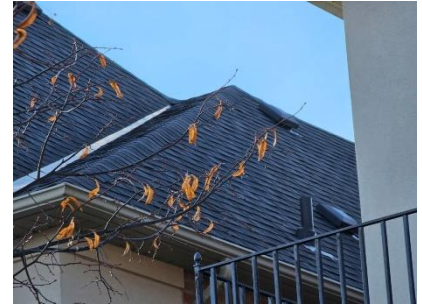
Pic. 3: Updated roof covering
