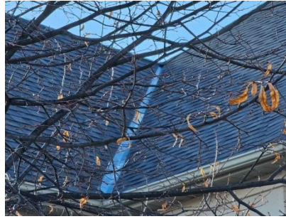
Pic. 2: Updated roof covering
