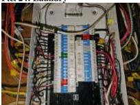
Pic. 27: 100 amp breaker panel with copper and aluminum wiring
