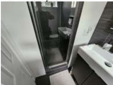
Pic. 22: Ground level bathroom
