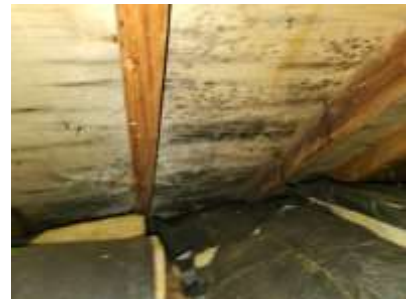
Pic. 9: Very small amount of staining/ possible surface mould growth in attic – area can just be cleaned
