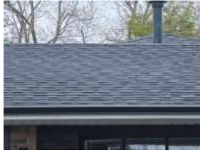
Pic. 2: Updated roof covering
