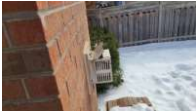
Pic. 4: Repaired fireplace vent
