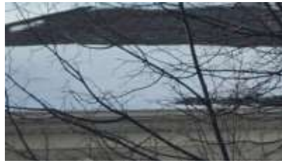
Pic. 2: Roof covering
