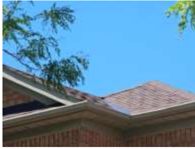
Pic. 2: Roof covering
