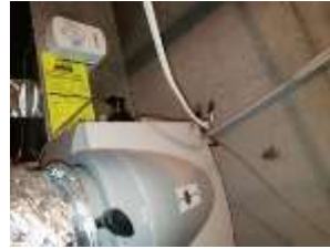
Pic. 27: Open live wire needs to be secured in a proper junction box
