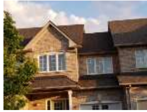
Pic. 2: Updated roof covering
