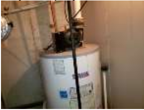
Pic. 25: Hot water tank
