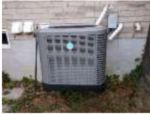
Pic. 5: AC unit
