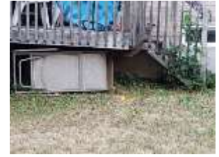
Pic. 4: Rear deck sagging, repair as necessary
