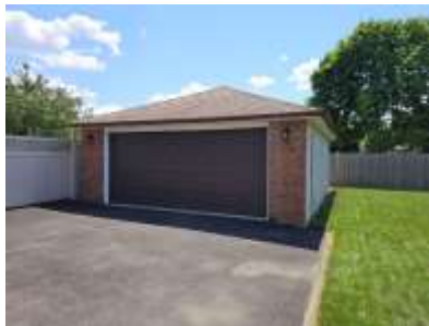
Pic. 8: Detached garage
