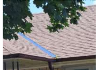
Pic. 3: Updated roof covering
