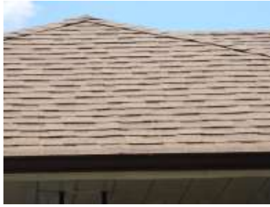
Pic. 2: Updated roof covering
