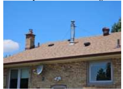
Pic. 6: Rear roof covering
