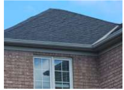
Pic. 3: Updated roof covering
