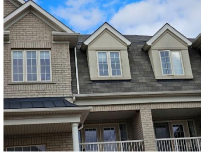
Pic. 2: Roof covering
