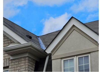
Pic. 3: Roof covering
