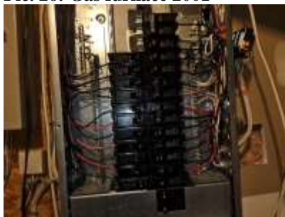
Pic. 29: 100 amp breaker panel
