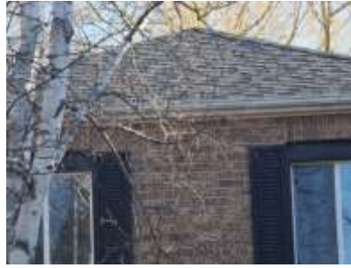
Pic. 2: Updated roof covering
