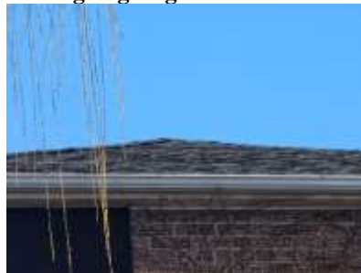
Pic. 11: Update roof covering
