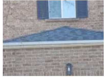
Pic. 3: Updated roof covering
