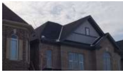
Pic. 2: Roof covering
