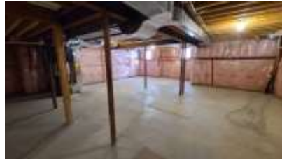
Pic. 26: Unfinished basement
