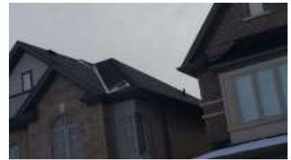
Pic. 3: Roof covering
