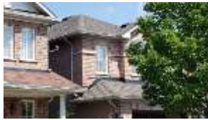
Pic. 2: Updated roof covering
