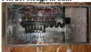
Pic. 30: 100 amp breaker panel with all copper wire
