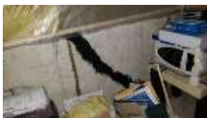
Pic. 29: Repaired foundation crack
