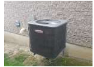
Pic. 4: AC unit 2008
