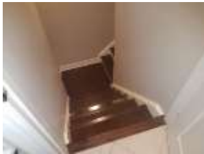
Pic. 29: Handrail needed for basement stairwell
