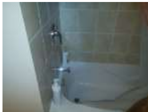
Pic. 38: Basement bath
