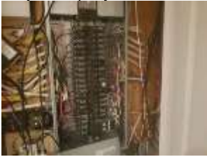
Pic. 41: 200 amp breaker panel with all copper wire
