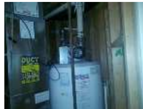
Pic. 39: Rental hot water tank
