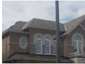
Pic. 2: Roof covering
