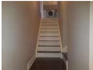
Pic. 30: Handrail needed for basement stairwell
