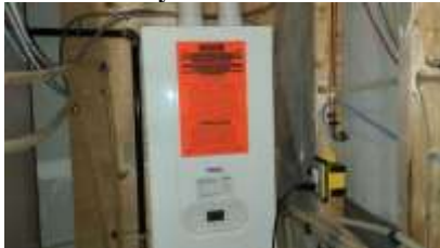
Pic. 25: Tankless hot water boiler 2018
