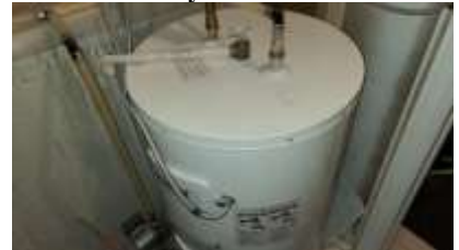
Pic. 27: Supplemental hot water tank for furnace
