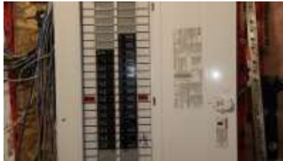
Pic. 29: 150-amp breaker panel
