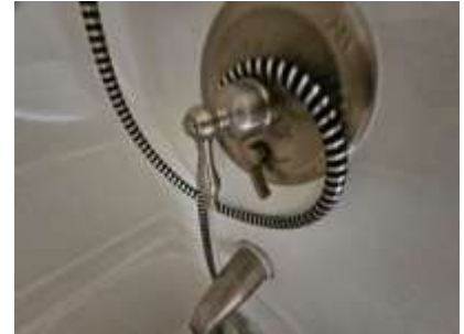
Pic. 24: Shower water diverter seized in shower position
