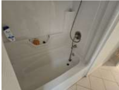
Pic. 23: 2 nd floor bath
