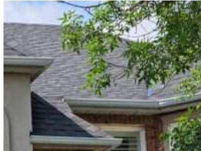
Pic. 2: Updated roof covering
