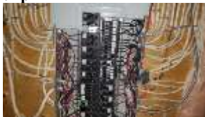
Pic. 45: 100 amp breaker panel
