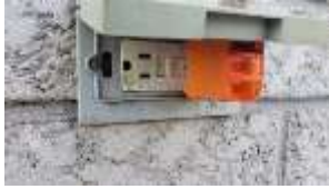
Pic. 5: Rear GFCO defective
