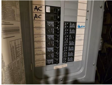
Pic. 32: 100 amp breaker panel
