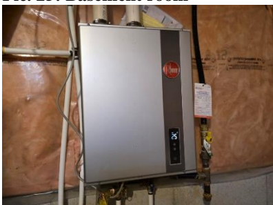
Pic. 28: Tankless hot water boiler 2024
