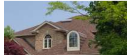
Pic. 3: Updated roof covering
