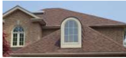
Pic. 2: Updated roof covering
