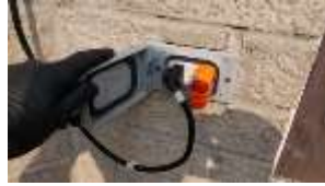
Pic. 6: Rear GFCI needs replacement
