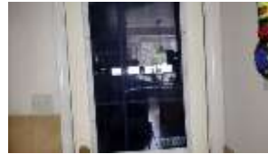
Pic. 31: Garage entry door not fire rated (glass insert) and requires an auto closer
