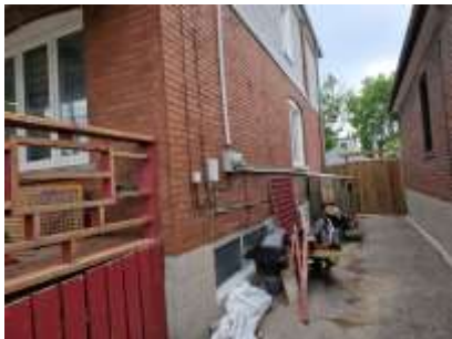
Pic. 4: Side view
