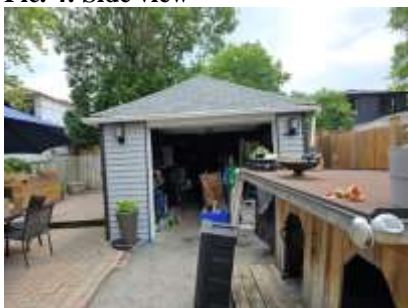
Pic. 7: Detached garage
