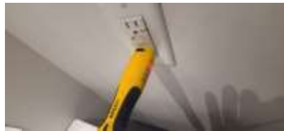
35: No grounding on bathroom GFCI outlet
