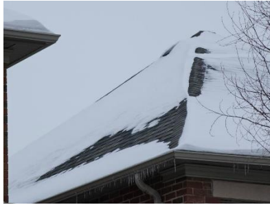
Pic. 2: Visible roof covering
