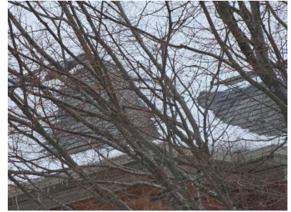
Pic. 3: Visible roof covering
