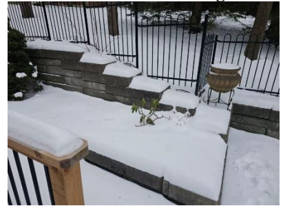
Pic. 6: Retaining walls
