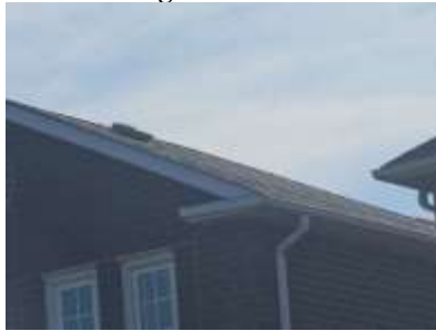
Pic. 5: Roof covering
