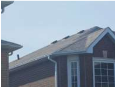
Pic. 4: Roof covering
