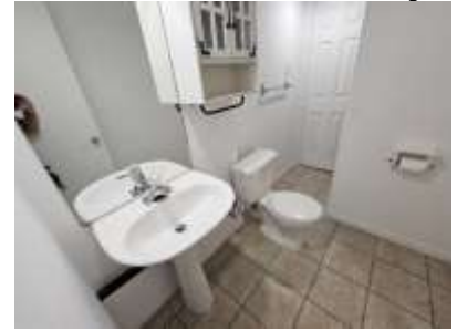
Pic. 48: Basement bathroom
