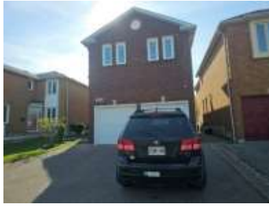
Pic. 2: Garage view
