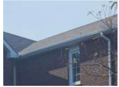
Pic. 3: Roof covering
