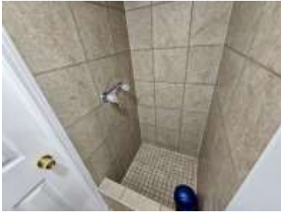
Pic. 49: Basement bathroom
