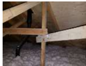
Pic. 15: Small amount of staining on sheathing, clean accordingly if necessary
