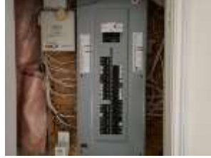
Pic. 39: 200 amp breaker panel
