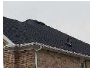
Pic. 3: Roof covering
