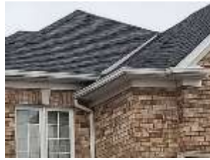
Pic. 2: Roof covering
