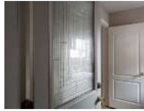
Pic. 11: Proper fire rated entry door for garage recommended
