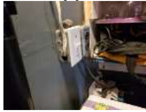
Pic. 10: Handyman / extension cord wiring needs review and correction
