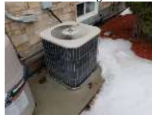
Pic. 7: AC unit 2002
