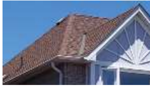
Pic. 2: Updated roof covering
