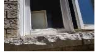
Pic. 4: Wood window frames need painting
