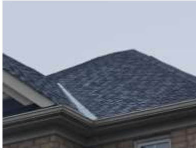
Pic. 2: Updated roof covering
