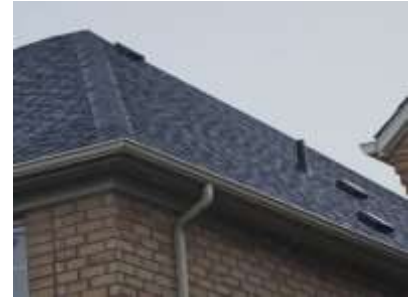
Pic. 3: Updated roof covering
