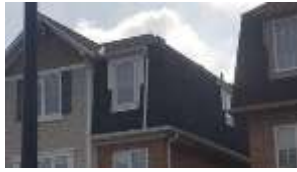
Pic. 2: Roof covering
