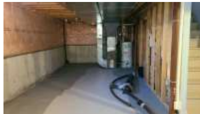
Pic. 29: Unfinished basement
