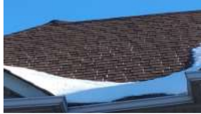
Pic. 2: Visible roof covering
