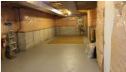
Pic. 28: Unfinished basement
