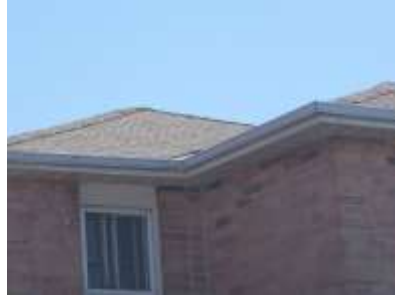
Pic. 2: Roof covering
