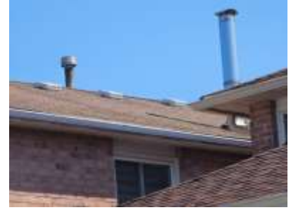
Pic. 3: Roof covering
