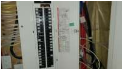
Pic. 43: 200 amp breaker panel
