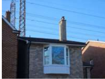
Pic. 2: Updated roof covering
