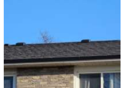
Pic. 6: Updated roof covering
