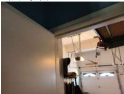
Pic. 7: Auto closer needed for garage entry door
