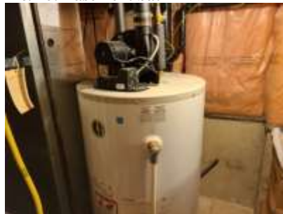
Pic. 29: Hot water tank
