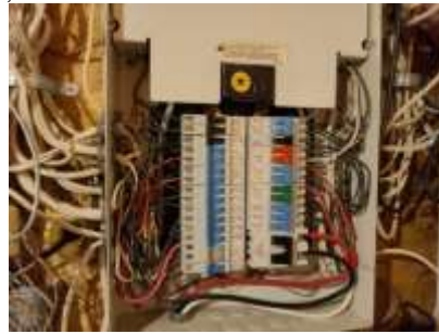
Pic. 32: 100 amp electrical panel
