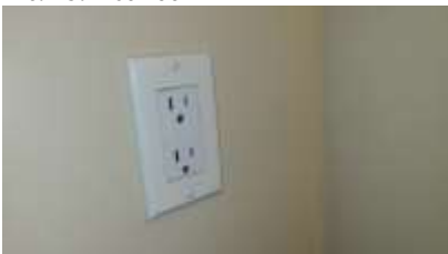
Pic. 31: Bathroom outlet should be GFCI protected
