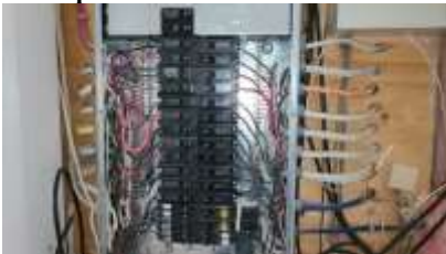
Pic. 34: 100 amp breaker panel
