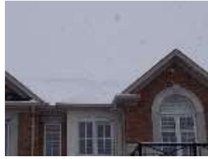
Pic. 2: Snow covered roof covering
