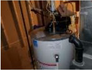
Pic. 29: New hot water tank
