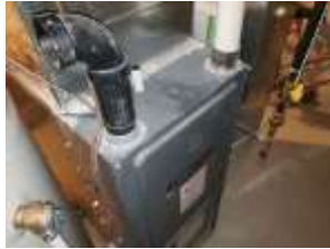
Pic. 30: Original gas furnace
