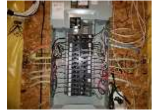
Pic. 32: 100 amp breaker panel
