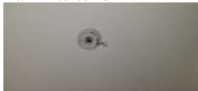
Pic. 17: Missing smoke detector on 2nd floor
