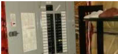
Pic. 31: 100-amp breaker panel
