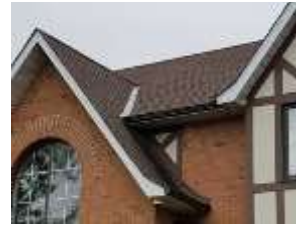
Pic. 3: Roof covering
