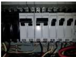
Pic. 37: One breaker oversized for wire size
