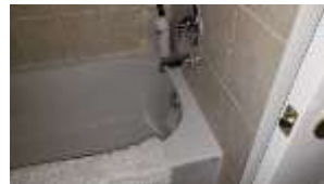
Pic. 15: 2 nd floor bath
