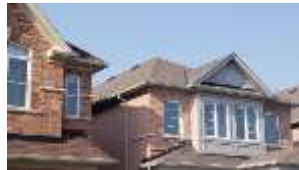
Pic. 2: Original roof covering
