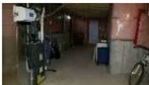
Pic. 25: Unfinished basement
