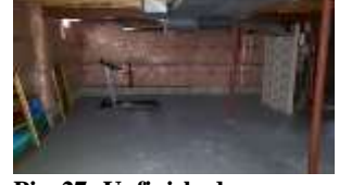
Pic. 27: Unfinished basement
