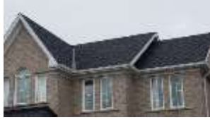
Pic. 2: Roof covering
