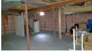
Pic. 28: Unfinished basement
