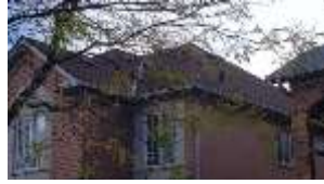
Pic. 2: Roof covering
