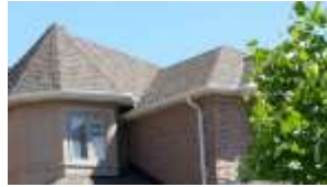
Pic. 2: Roof covering
