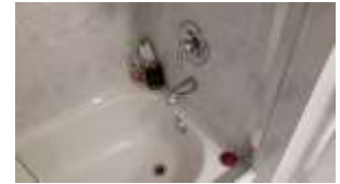
Pic. 16: Shower/ tub water spout diverter seized
