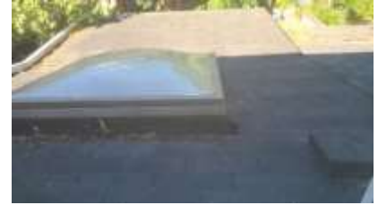
Pic. 6: Flat roof area
