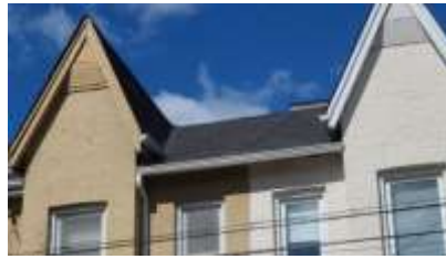
Pic. 2: Roof covering
