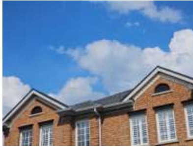
Pic. 2: Updated roof covering
