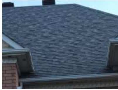
Pic. 2: Updated roof covering
